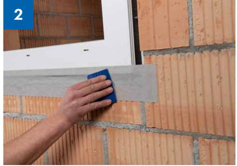
> Rub the adhesive tapes on well using the Ampacoll® Pressly press-on aid.
