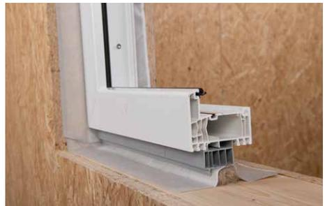
> Stick Ampacoll® Fenax DS for alternating bonding to the inside and outside of the window frame, then press on well. Create corner loops: approx. 1.5×joint width. Insulate joints ensuring there are no cavities. Left: without window connection profile (FBA). Right: with FBA. **Note:** Observe the design of the window sill base, see pages 17–19 second sealing layer / window sill base.
