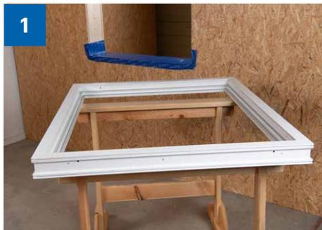
> Position and clean the window frame. Here we started with the inside.
