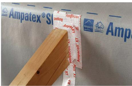
Adhesion to corners and angles – 30 mm on one side, and 30 mm on the other
