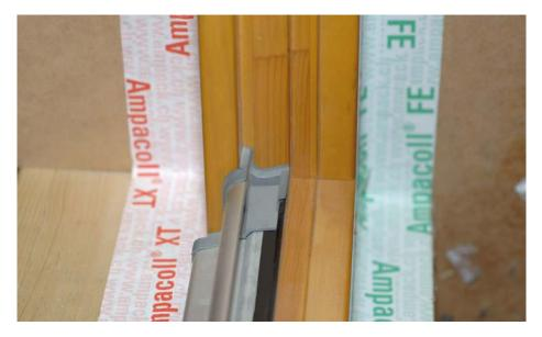
Window installation – 12 mm for sticking the adhesive tape to the window frame, then the rest (48 mm) on the embrasure
