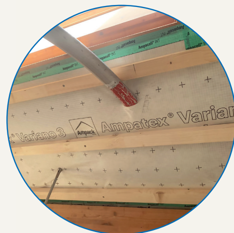
Ampatex® Variano 3 extra: ideal for injection insulation due to its high tear resistance.
